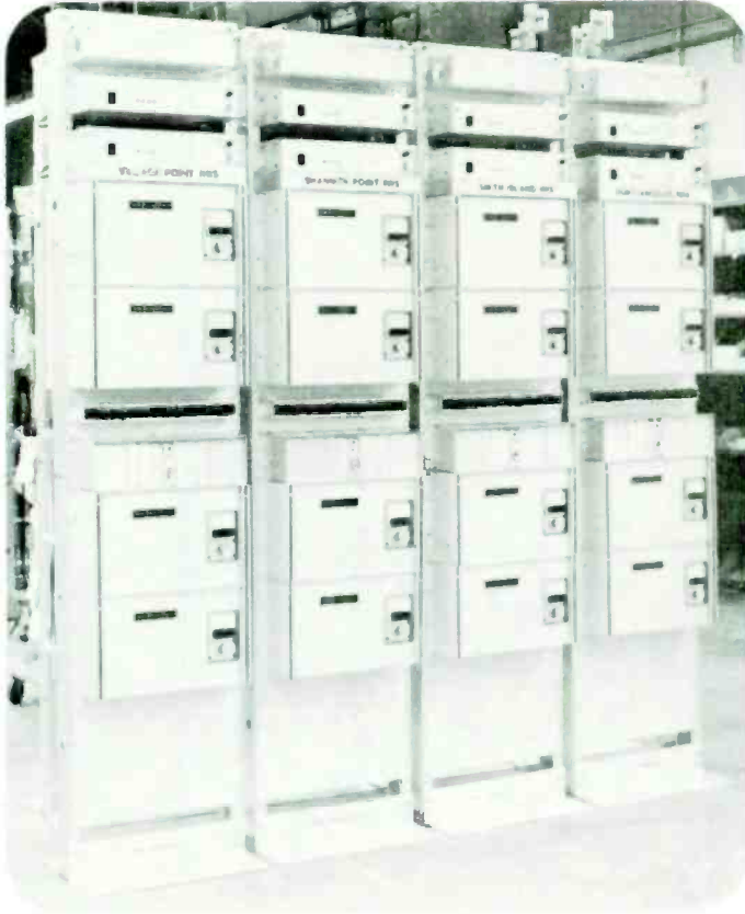
Typical FV8F protected IF repeaters
